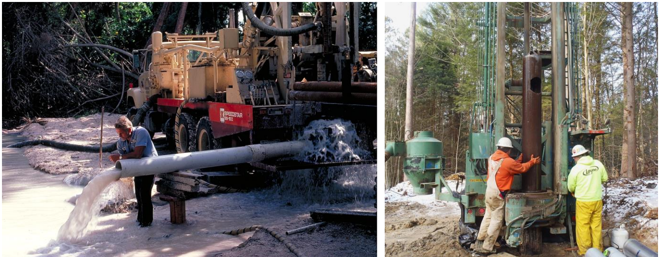
Figure 16.28 Well development methods. Left: Airlift, photo courtesy of Dr. Gerald Seaburn. Right: Bailer, photo courtesy of Mark Bauer.
