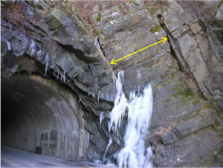
Figure 7.12 Frozen discharge of groundwater along margins of a 9-ft wide dike (denoted by arrows) and fractures in gneiss at the north portal to tunnel at Marys Rock in the Blue Ridge Mountains, located at mile marker 32.2 on Skyline Drive in Virginia.
