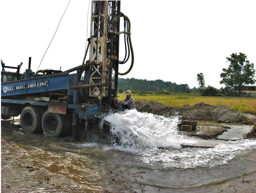
Figure 6.26 Development of a high yielding well in Michigan, completed in glacial sand and gravel. Photo courtesy of Jim Brode.
