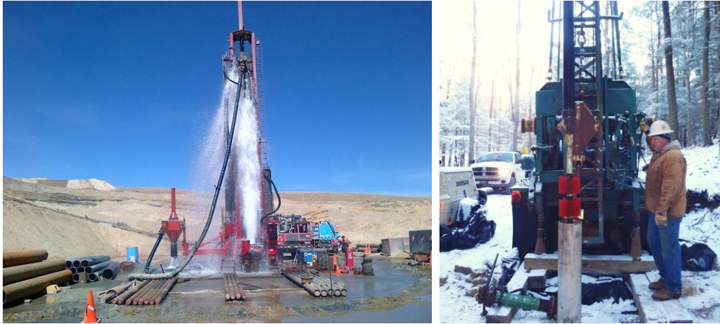
Figure 16.27 Well development methods. Left: Compressed air, photo courtesy of Dave Evans. Right: Wire brush, photo courtesy of Mark Bauer.
