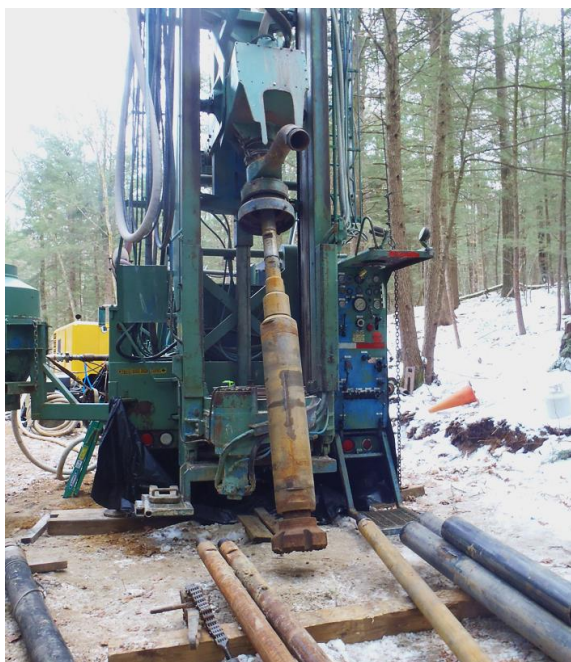
Figure 14.25 Rotary drill bit on a dual rotary drill rig used to install a monitoring well in a karst aquifer in New York state, U.S. Courtesy of Mark Bauer.
