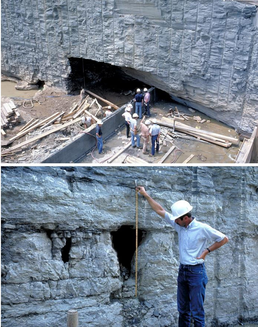
Figure 7.17 Cavities of varying size discovered at a deep (seen dewatered here) construction site in Hartsville, Tennessee. Photographs by George Sowers; printed with kind permission of Francis Sowers.
