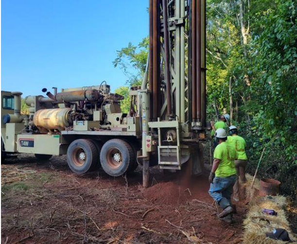
Figure 14.26. Air rotary drilling during a monitoring well installation at a coal ash landfill in Eastern United States. Courtesy of Ted Wilson.
