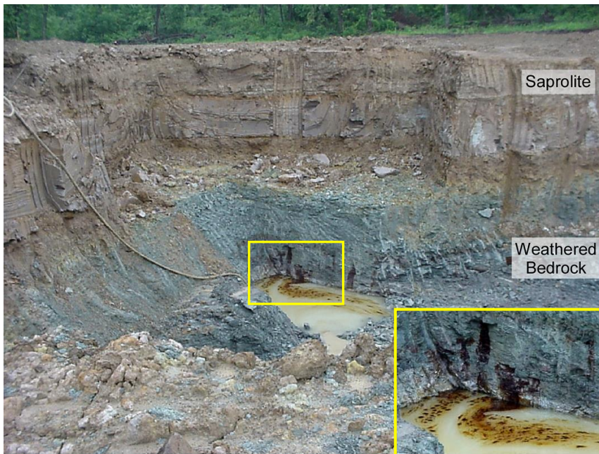
Figure 7.10 Photograph taken during the excavation phase of a coal tar remediation project shows distinctive reddish-brown mottling in a weathered siltstone where oil seeps occur along shallow dipping (3-4 degrees) bedding plane fractures. Courtesy of Peter Thompson; photograph by Leo E. Arbaugh, Jr. of the U.S. Army Corps of Engineers.
