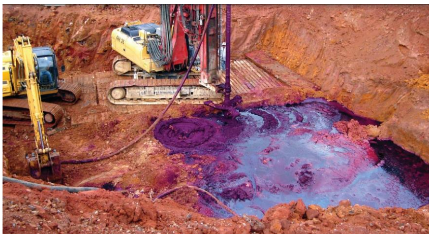
Figure 13.22 Direct permanganate mixing with contaminated regolith soil over fractured metamorphic rock near Atlanta, GA. Photo courtesy of Rick Marotte, Law Engineering and Environmental Services, Inc.
