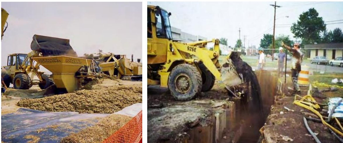
Figure 13.27 Left : Installation of ZVI PRB at a U.S. Coast Guard facility using a one-pass trencher. Right : Coarse-grained ZVI being placed in a trench for a PRB. Courtesy of ITRC, 2011. Copyright ITRC; acknowledgement required for further use.
