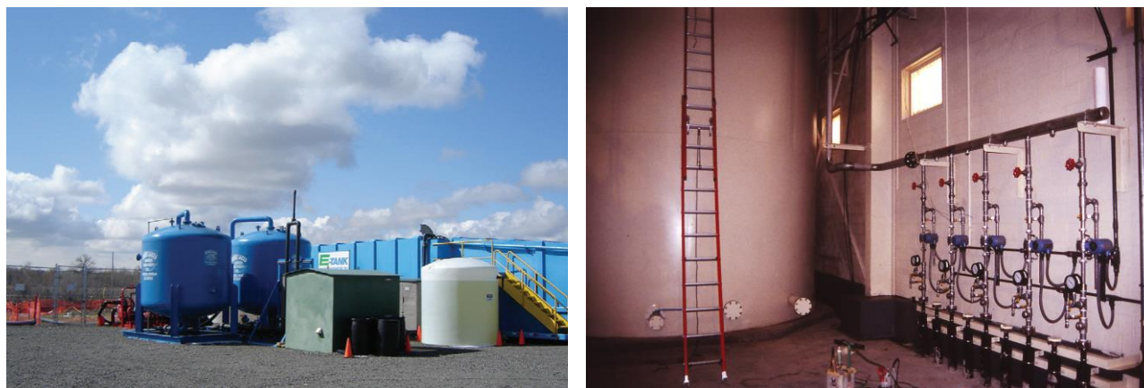
Figure Left: Outdoor treatment facilities. From EPA-542-F-21-021. In public domain. Right : Control room for a P&T system with five extraction wells; treatment tank is on the left.
