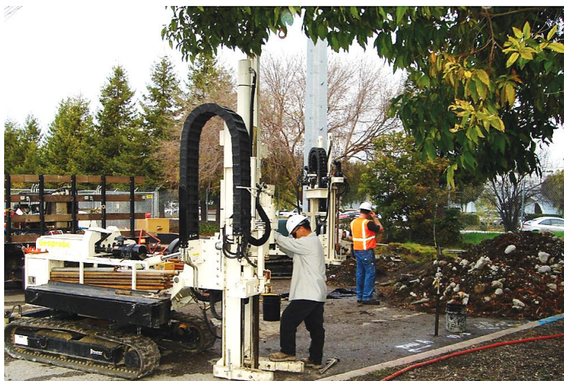
Figure 13.25 Biostimulation, or injection of vegetable oil underground to improve conditions for bioremediation. From EPA-542-F-21-004; in public domain.
