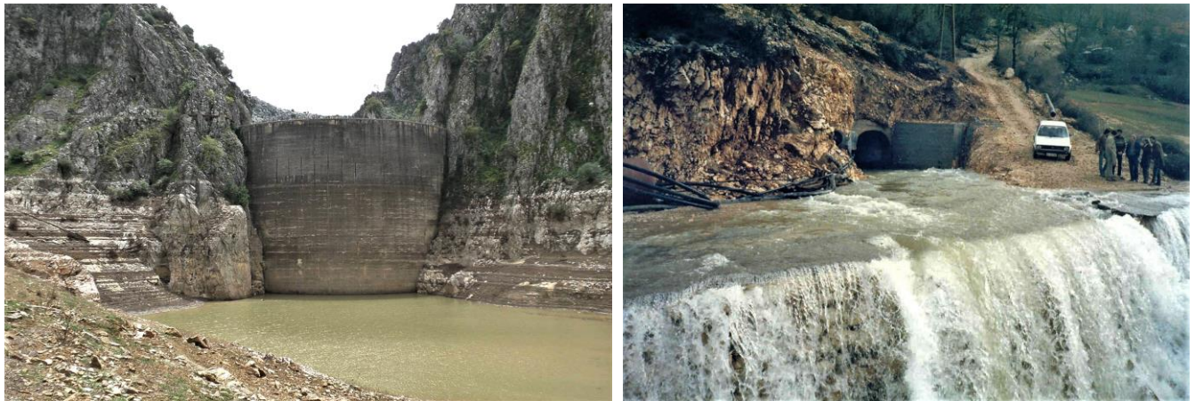
Figure 7.15 Left: Montejaque Dam in the Sierra de Grazalema, Spain, was abandoned before the Second World War because of large losses of water from the reservoir and at the dam site through numerous sinks and other karst features. This arc dam on the river Compobuche-Guadares, a tributary of the Guadiaro river, is 83.75 m high with an 84-m long crest. After heavy rains, the reservoir behind the dam fills with water only to lose it soon after rains stop. Right: Hydrotechnical tunnel in Dabarsko Polje, Herzegovina, flooded during construction. Photographs courtesy of Petar Milanović.
