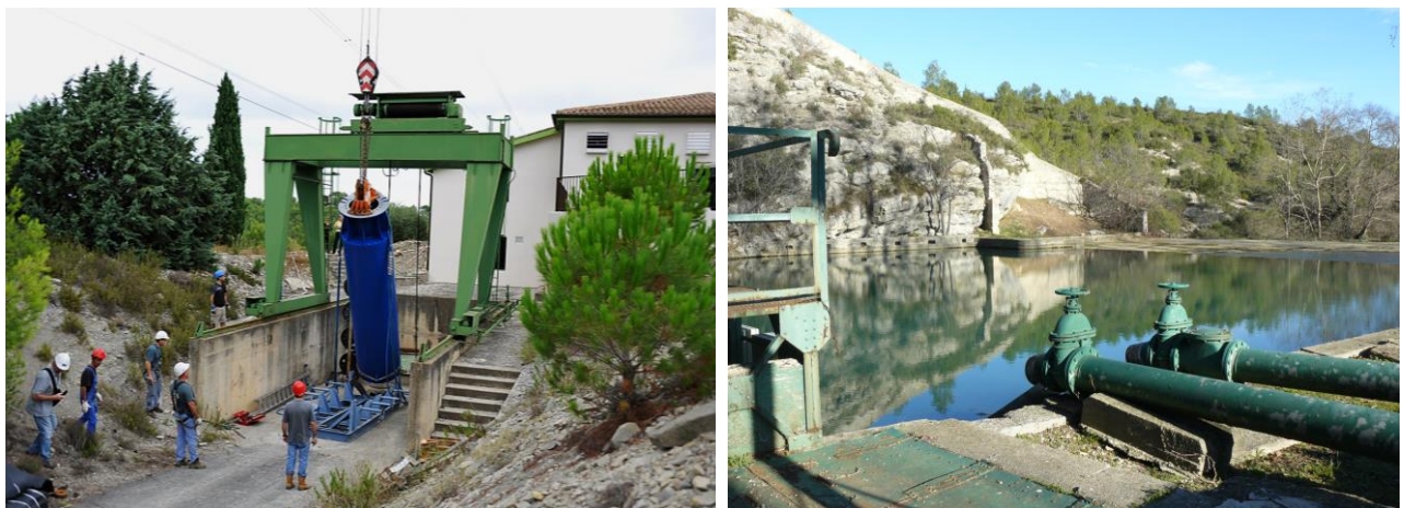
Figure 16.43 Left : Replacement of a high-capacity submersible pump in one of the extraction wells at the Spring of River Lez (Source du Lez) utilized for water supply of Montpellier, France. Photo courtesy of Jean Michel Valéry. Right : Old pumping installation at the spring. Photo courtesy of Arnaud Vestier, Service des Eaux, city of Montpellier.
