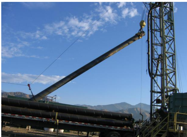
Figure 16.23 Large-diameter casing being installed in a deep production well in Arizona. Photo courtesy of Adrian Ezeagy.
