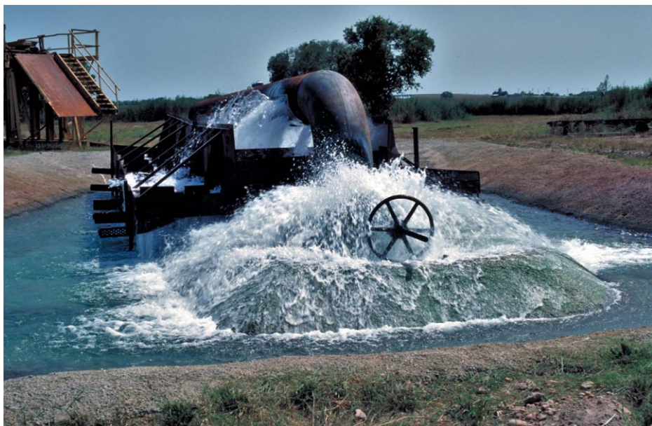
Figure 7.30 The highest capacity drilled well in the world, capable of sustained pumping of 40000 gallons per minute ( 2.5 \text{ m}^3/\text{sec} ), located on the Ron Pucek's Catfish Farm near San Antonio, Texas. Photo copyright by Gregg Eckhardt; printed with kind permission.
