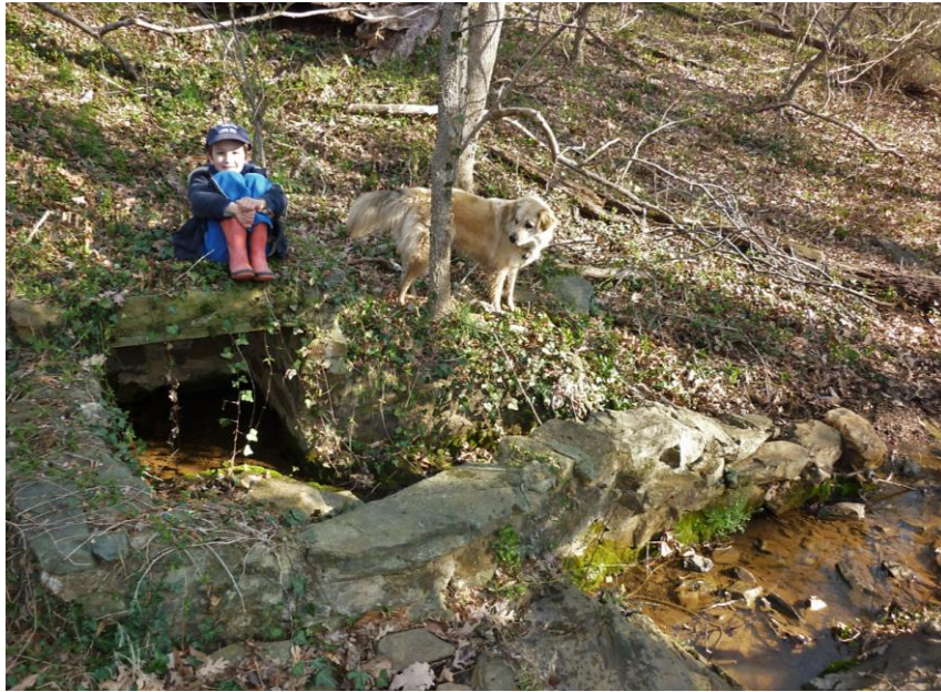
Figure 7.11 Simple capture of a low yielding but permanent spring tapped for water supply of a farmhouse before the Civil War. Many similar springs are still used as sources of potable water in the Virginia's Piedmont physiographic province, although drilled wells are now the main form of private water supply in the region.
