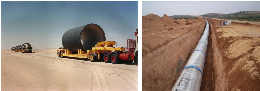
Figure 16.20 For the construction of Great Man-Made River project in Libya, prestressed concrete cylinder pipes 4 meters in diameter and 7.5 meters long, weighing up to 80 tons, were brought to the excavation sites using a fleet of some 128 specially designed transporters. Each pipe was buried in a trench approximately seven meters deep, excavation of which required the removal of some 100,000 cubic meters of material each working day. Excavation was carried out by large hydraulic excavators fitted with 7.6 m 3 buckets. Left photo courtesy of Jaap Berk, The Netherlands; in public domain. Right photo courtesy of https://alk3r.wordpress.com/2017/07/04/the-great-man-made-river-of-libya/ .
