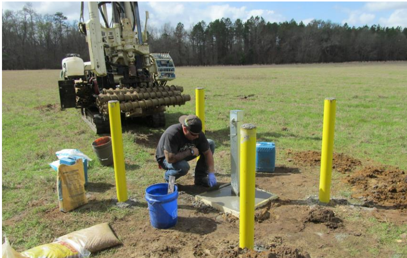
Figure 14.29 Typical completion of a monitoring well showing riser pipe, concrete surface pad, and bumper guards for surface protection. Hollow stem auger drill rig is in the background. Photo courtesy of Dawit Yifru.
