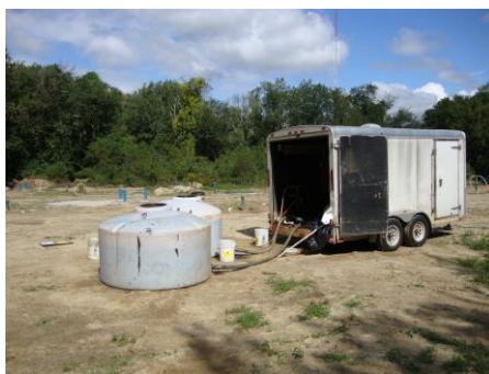
Figure 13.23 Left : Installation of a horizontal injection well in a gravel-filled trench design to inject 4% sodium-permanganate solution into a source zone in southern New England. Right : ISCO treatment area. The trailer contains a pump to inject the permanganate under pressure. Courtesy of Woodard & Curran, Inc.
