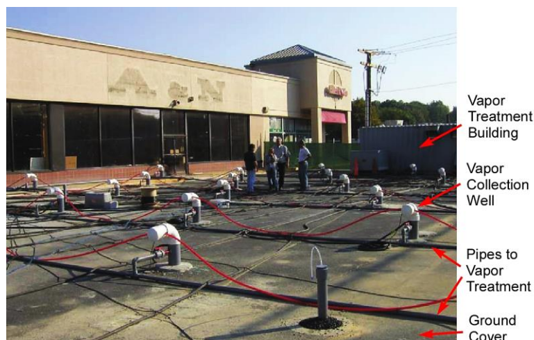
Figure 13.24 ERH system for remediation of contaminated soil and groundwater. Note that the surface was paved to prevent cooling effects of aerial recharge. From EPA-542-F-21-016; in public domain.
