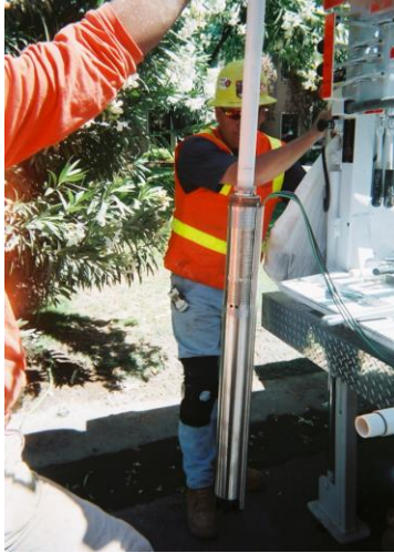
Figure 15.32 Installation of a submersible pump for an aquifer pumping test. Photo courtesy of Adrian Ezeagy.
