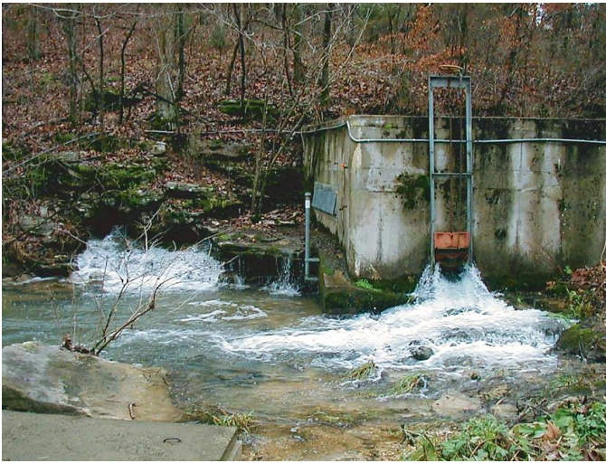
Figure 16.40 Photograph of the outflow from the spring box of Hughes Spring near Zack, Arkansas. Hughes Spring supplies water for the city of Marshall, Arkansas, and the surrounding area. The mean annual discharge for Hughes Spring was 2.9 and 5.2 cubic feet per second for water years 2001 and 2002, respectively. Tritium data for Hughes Spring indicate that the discharge water is a mixture of recent recharge and sub-modern water (recharged prior to 1952). Photograph by Joel Galloway, USGS, from Galloway, 2004; in public domain.
