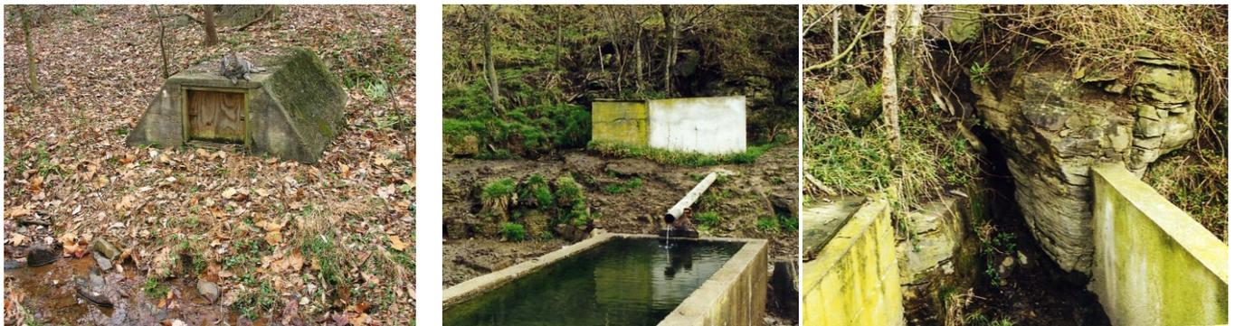
Figure 16.36 *Left*: Abandoned capture of a spring historically used for water supply of a pre-civil war farmhouse in Rixeyville, Virginia. Two right photographs show capture of a fracture spring utilized for watering cattle on a farm near Saltville, Virginia.
