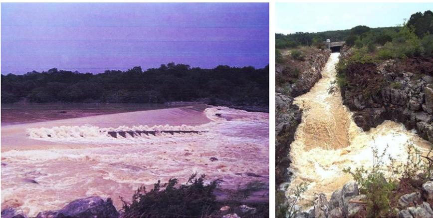
Figure 16.47 *Left:* Edwards Aquifer recharge dam on Seco Creek, Texas. *Right:* During the flood events like the one shown on the left, part of the flood water is diverted towards the Valdina sink via artificial channel incised into the Edwards Limestone. Photographs courtesy of Edwards Aquifer Authority. See also Figure 7.38 in Lecture 7, and [www.edwardsaquifer.net/intro.html](http://www.edwardsaquifer.net/intro.html).
