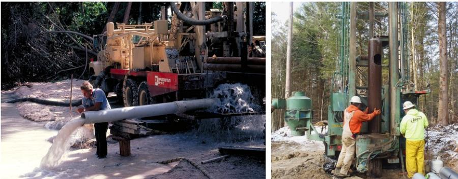
Figure 16.24 Well development methods. *Left:* Airlift, photo courtesy of Dr. Gerald Seaburn. *Right:* Bailer, photo courtesy of Mark Bauer.
