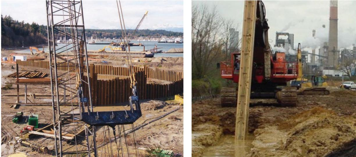
Figure 13.26 *Left*: Installation of sheet piling. *Right*: Construction of a slurry wall.
