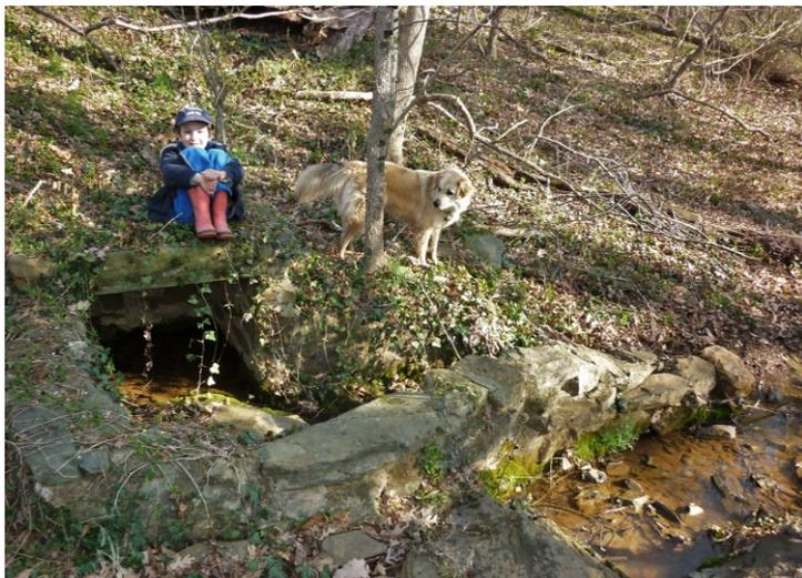
Figure 7.9 Simple capture of a low yielding but permanent spring tapped for water supply of a farmhouse before the Civil War. Many similar springs are still used as sources of potable water in the Virginia's Piedmont physiographic province, although drilled wells are now the main form of private water supply in the region.
