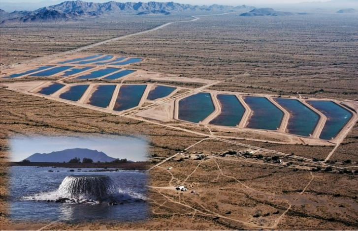
Figure 16.46 Tonopah Recharge Site, Central Arizona Project. Inset: Delivery of recharge water to one of the basins. Photographs courtesy of Philip Fortnam, Central Arizona Project.
