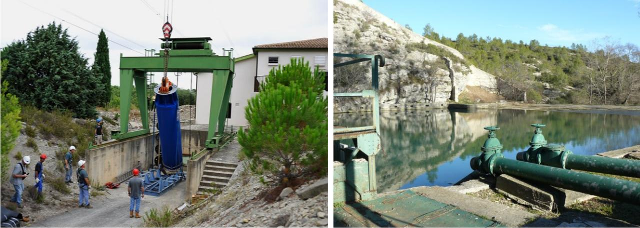
Figure 16.43 *Left*: Replacement of a high-capacity submersible pump in one of the extraction wells at the Source of River Lez (Source du Lez) utilized for water supply of Montpellier, France. Photo courtesy of Jean Michel Valéry. *Right*: Old pumping installation at the spring. Photo courtesy of Arnaud Vestier, Service des Eaux, city of Montpellier.
