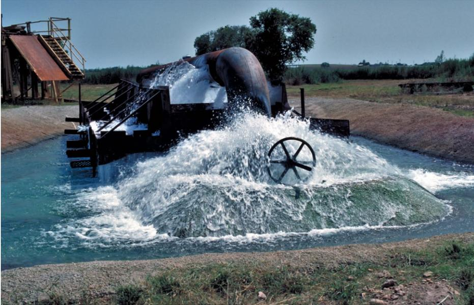
Figure 7.28 The highest capacity drilled well in the world, capable of sustained pumping of 40000 gallons per minute ( $2.5 \text{ m}^3/\text{sec}$ ), located on the Ron Pucek's Catfish Farm near San Antonio, Texas. Photo copyright by Gregg Eckhardt; printed with kind permission.
