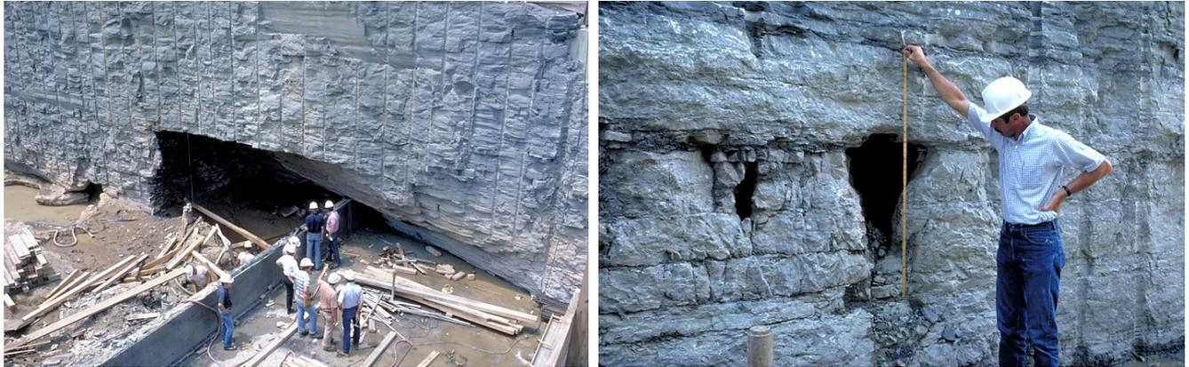
Figure 7.15 Cavities of varying size discovered at a deep (seen dewatered here) construction site in Hartsville, Tennessee. Photographs by George Sowers; printed with kind permission of Francis Sowers.
