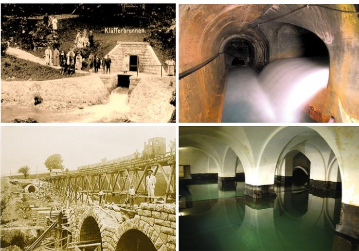
Figure 16.4 *Top left:* Historic picture of the entrance no. 11 and overflow of the Kläffer Spring (around 1910). *Top right:* Partially flooded overflow gallery of the Kläffer Spring underground capture. *Lower left:* Construction of an aqueduct of the Second Vienna Water Main. *Lower right:* One of the city waterworks’ storage reservoirs at Vienna Rosenhügel with a volume of 120,500 m<sup>3</sup>. Photos courtesy of Lukas Plan, Gerhard Kuschnig, and Hermann Stadler.
