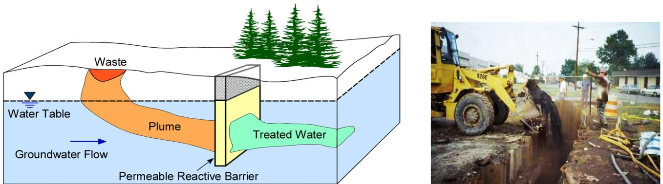
Figure 13.25 *Left*: Example of a plume being treated by a permeable reactive barrier (PRB). Modified from U.S. EPA, 1998b, in public domain. *Right*: Coarse-grained ZVI being placed in a trenched PRB. Courtesy of ITRC, 2011. Copyright ITRC; acknowledgement required for further use.
