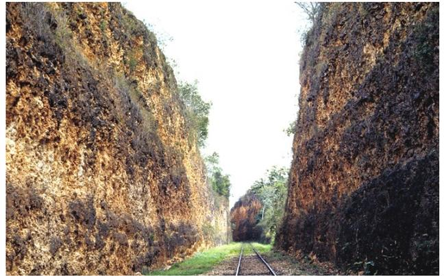
Figure 7.34 Dry railroad cut in limestone, Dominican Republic, showing no signs of perched epikarst zone. Photographs by George Sowers, printed with kind permission of Francis Sowers.
