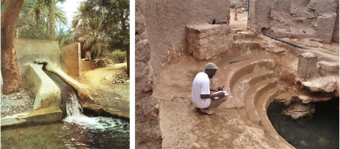
Figure 16.34 *Left*: Capture of Hammam Sharqi Spring in the Sultanate of Oman. Part of water (seen here) from this hot spring ( $41^{\circ}\text{C}$ ) is used for irrigation. Chebaane et. all (1994). *Right*: Ancient spring intake Taalex Laasqoray Xudun, still actively used by local population; Sool Plateau-Sanaag, Puntland Province, Somalia. Courtesy of Zoran Stevanović.
