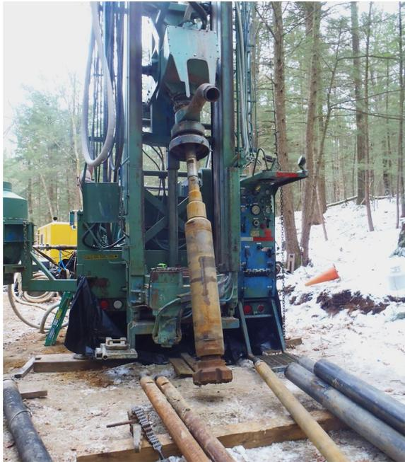
Depending on the site-specific conditions, the following drilling methods may be suitable for the installation of environmental monitoring wells (see also Section 14.4): hollow stem auger (HAS), sonic (rotasonic), air rotary (which can be supplemented with down-the-hole (DTH) percussion hammers driven by the air stream to rapidly penetrate bedrock materials), and cable tool. In all cases, the preferred methods are those that case the hole during drilling.
