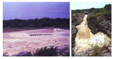
Figure 16.47 *Left*: Edwards Aquifer recharge dam on Seco Creek, Texas. *Right*: During the flood events like the one shown on the left, part of the flood water is diverted towards the Valdina sink via artificial channel incised into the Edwards Limestone. Photographs courtesy of Edwards Aquifer Authority. See also Figure 7.38 in Lecture 7, and www.edwardsaquifer.net/intro.html.
