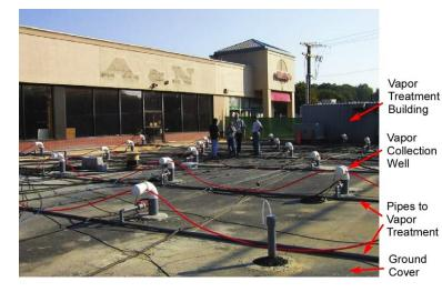
Figure 13.23 ERH system for remediation of contaminated soil and groundwater. Note that the surface was paved to prevent cooling effects of aerial recharge. From EPA-542-F-21-016, in public domain.
