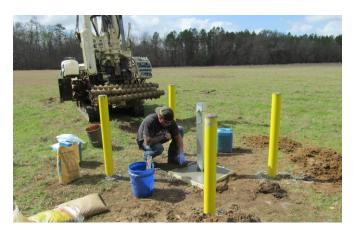
Figure 14.27 Typical completion of a monitoring well showing riser pipe, concrete surface pad, and bumper guards for surface protection. Hollow stem auger drill rig is in the background. Photo courtesy of Dawit Yifru.
