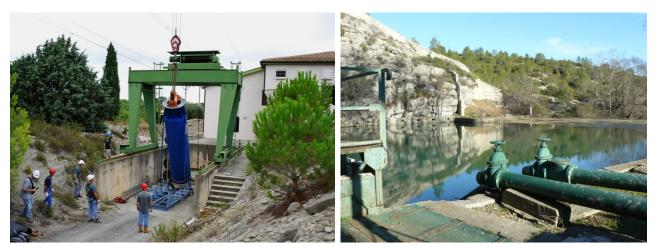
Figure 16.43 *Left*: Replacement of a high-capacity submersible pump in one of the extraction wells at the Source of River Lez (Source du Lez) utilized for water supply of Montpellier, France. Photo courtesy of Jean Michel Valéry. *Right*: Old pumping installation at the spring. Photo courtesy of Arnaud Vestier, Service des Eaux, city of Montpellier.
