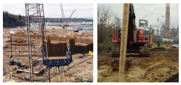
Figure 13.26 *Left*: Installation of sheet piling. *Right*: Construction of a slurry wall. From EPA-542-F-21-026, in public domain.
