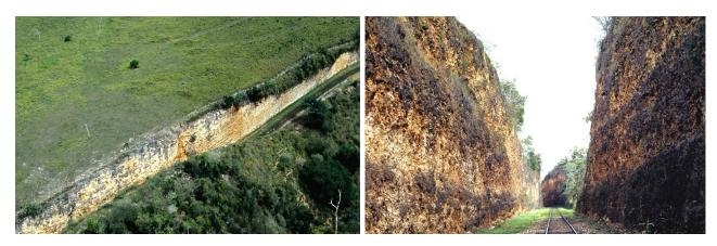
Figure 7.34 Dry railroad cut in limestone, Dominican Republic, showing no signs of perched epikarst zone. Photographs by George Sowers, printed with kind permission of Francis Sowers.
