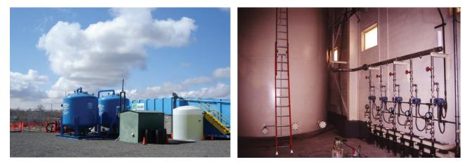
Figure 13.16 Left: Outdoor treatment facilities. From EPA-542-F-21-021. In public domain. *Right*: Control room for a P&T system with five extraction wells; extracted groundwater treatment tank is on the left.
