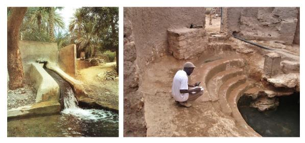
Figure 16.34 *Left*: Capture of Hammam Sharqi Spring in the Sultanate of Oman. Part of water (seen here) from this hot spring (41°C) is used for irrigation. Chebaane et. all (1994). *Right*: Ancient spring intake Taalex Laasqoray Xudun, still actively used by local population; Sool Plateau-Sanaag, Puntland Province, Somalia. Courtesy of Zoran Stevanović.
