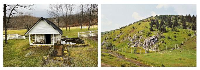
Figure 16.37 *Left*: Spring house built on top of an ascending spring at a historic plantation in Bath County, Virginia. The house also served as a food storage because of the cool air maintained by the spring water. *Right*: Spring-box type capture of the Lakomica spring issuing at the contact between fractured limestone and underlying low-permeable diabase. Fence around the spring area prevents access to the capture. The spring supplies drinking water to a town in western Serbia.
