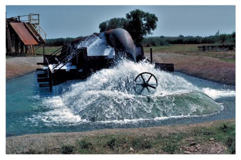
Figure 7.28 The highest capacity drilled well in the world, capable of sustained pumping of 40000 gallons per minute (2.5 m<sup>3</sup>/sec), located on the Ron Pucek's Catfish Farm near San Antonio, Texas. Photo copyright by Gregg Eckhardt; printed with kind permission.
