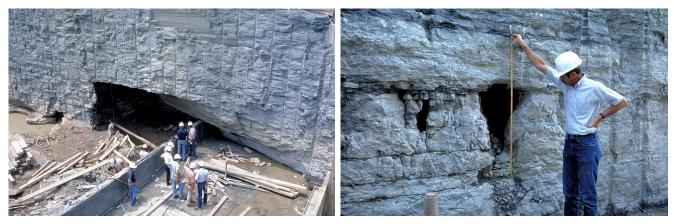
Figure 7.15 Cavities of varying size discovered at a deep (seen dewatered here) construction site in Hartsville, Tennessee. Photographs by George Sowers; printed with kind permission of Francis Sowers.
