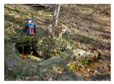
Figure 7.9 Simple capture of a low yielding but permanent spring tapped for water supply of a farmhouse before the Civil War. Many similar springs are still used as sources of potable water in the Virginia's Piedmont physiographic province, although drilled wells are now the main form of private water supply in the region.
