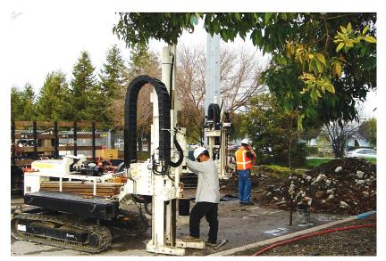
Figure 13.24 Biostimulation, or injection of vegetable oil underground to improve conditions for bioremediation. From EPA-542-F-21-004, in public domain.
