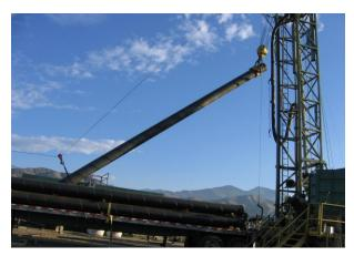
Figure 16.19 Large-diameter casing being installed in a deep production well in Arizona. Photo courtesy of Adrian Ezeagy.
