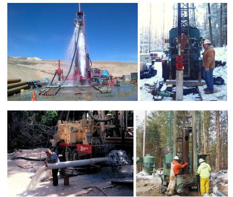
Figure 16.23 Well development methods. *Left*: Compressed air, photo courtesy of Dave Evans. *Right*: Wire brush, photo courtesy of Mark Bauer.
