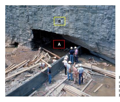
Figure 5.26 Cavity discovered below water table at a deep construction site (shown dewatered here) in Paleozoic limestone, Hartsville, Tennessee. Photo by George Sowers, printed with kind permission of Francis Sowers.
